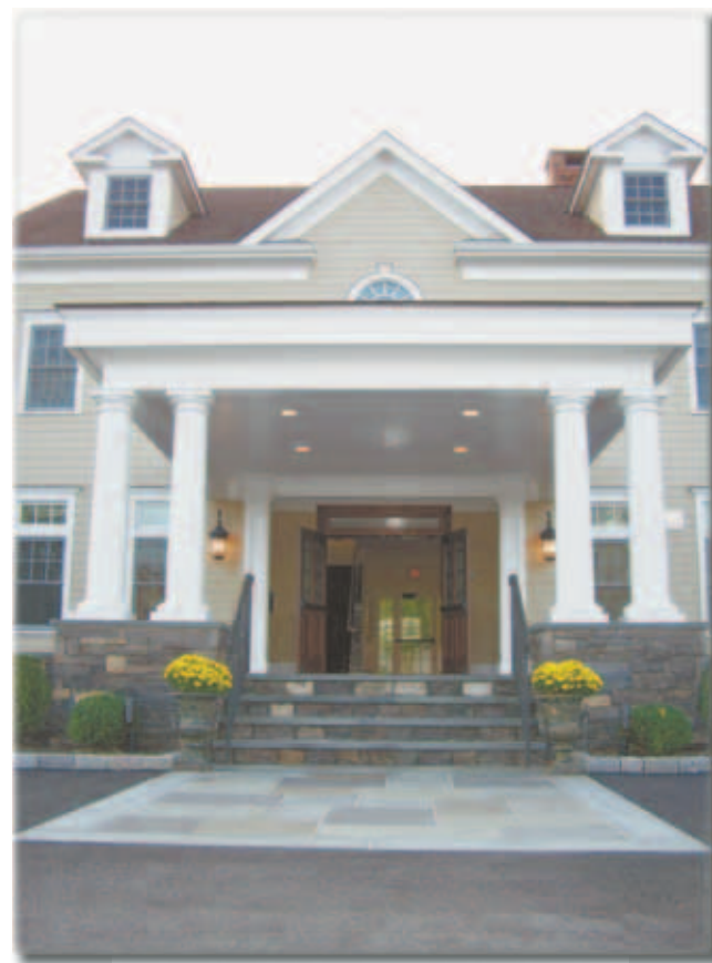
The Front Portico Entrance
