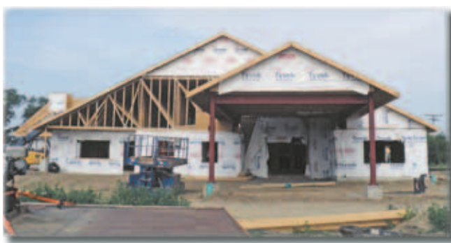
Elmwood Funeral Home under construction
