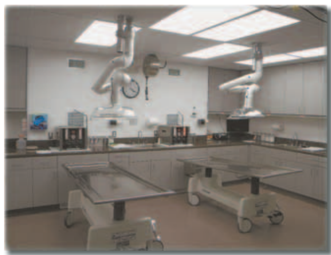
Preparation room with the new filtration introduced by DST.
