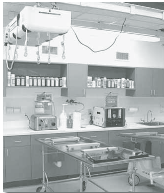
Foot-end View of Preparation Room
