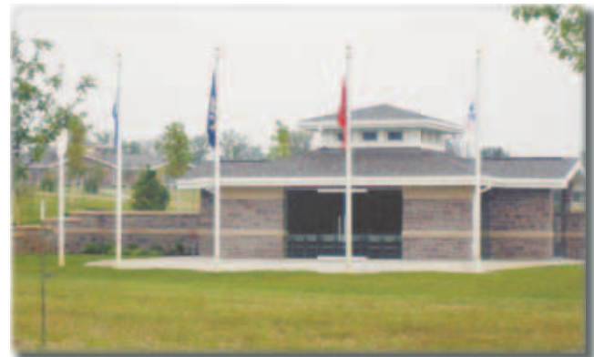
The committal service shelter at Iowa Veterans Cemetery with the administration building in the background.
