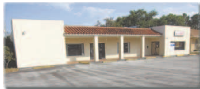
Vacant since mid-2009, the building had fallen into disrepair
