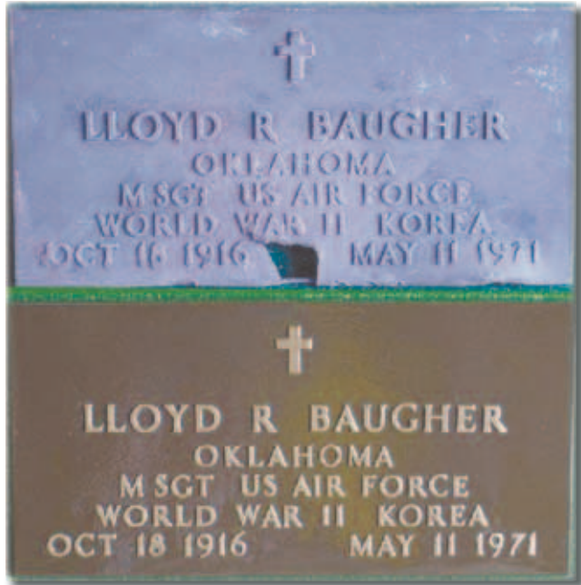
An example of American Memorial Restoration's work, a bronze plaque before and after restoration.
