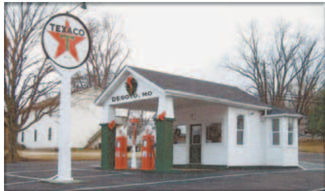
The DeSoto Texaco Station, before (top) and after renovation.
