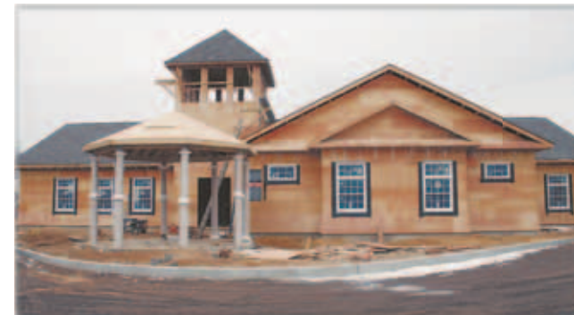
James Funeral Home's South Chapel in Construction
