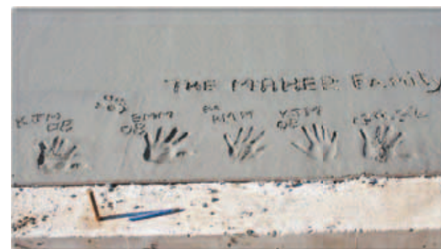
The family's handprints in the new cement.
