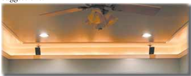
Rope lighting used with crown molding
